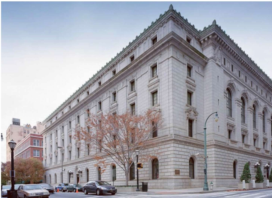
Elbert P. Tuttle Courthouse, Atlanta, home of the 11th Circuit Court of Appeals.
